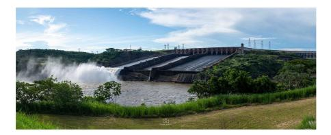
The dam's spillway is particularly impressive. When fully opened it can handle 10x the water flow as the record amount to go over Niagra Falls. This is an important safety feature. While much less known internationally than the Amazon, the Paraná River that it dams up is the second largest in South America so its important to be prepared for emergencies.
